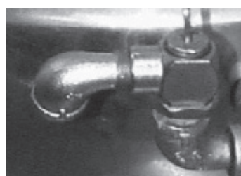
The open end of the pressure relief valve elbow must face downward.
