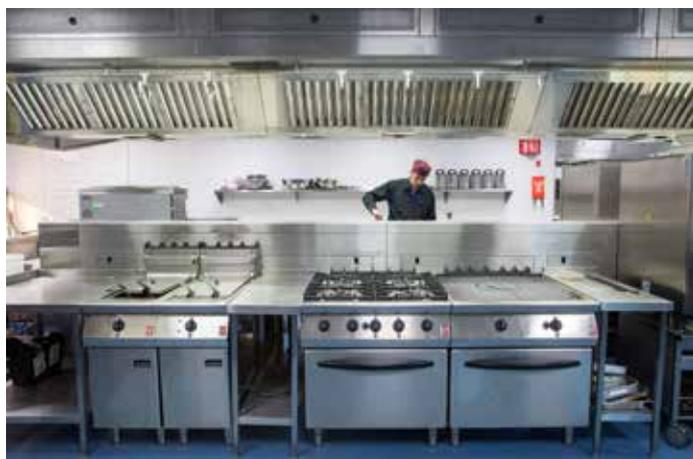
to clean. Both ranges have ovens capable of holding 2/1 Gastronorm trays, and have metal-to-metal door seals ensuring temperature is maintained in the oven, increasing efficiency. Fryers have advanced temperature control and automatic filtration to maintain oil quality for longer.
